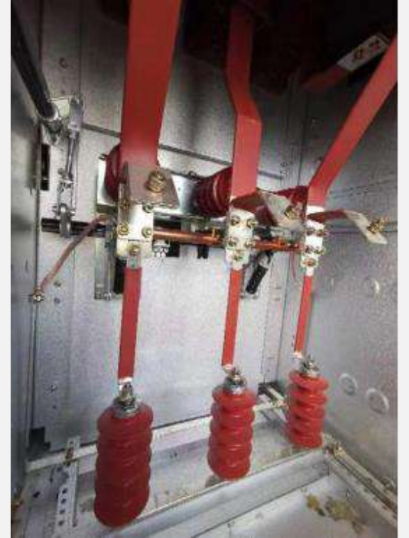
Earthing knife switch opening and closing device
