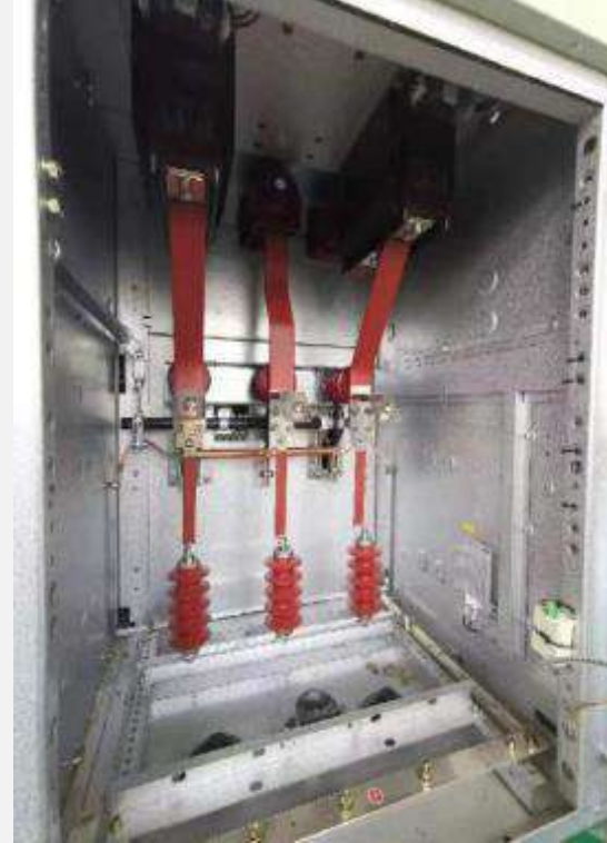
Earthing knife switch opening and closing device
