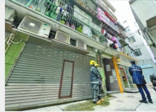
Three people died of suspected carbon monoxide poisoning in a unit near Banzhao Hall
